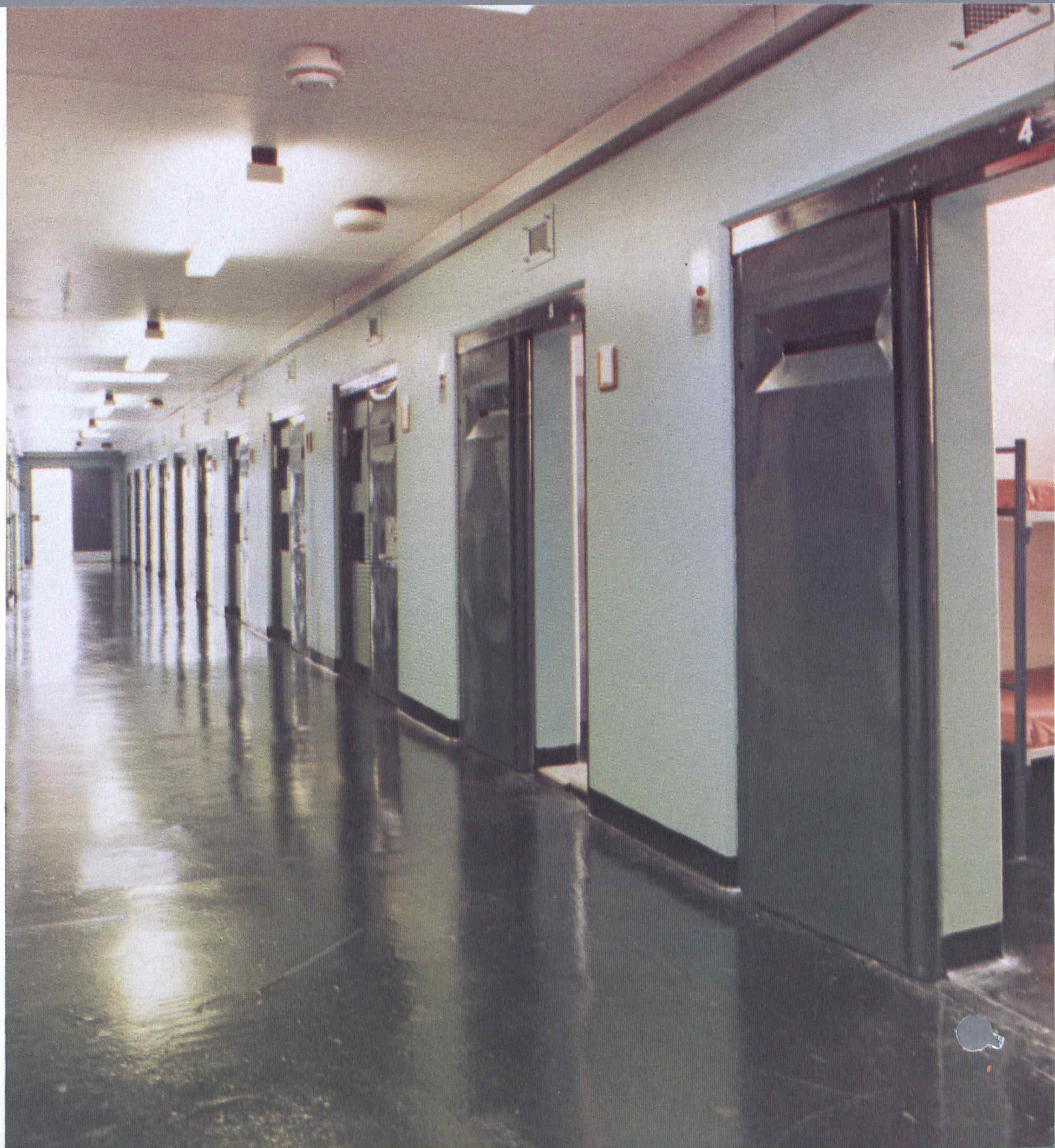
A corridor in a wing of an H-block.
