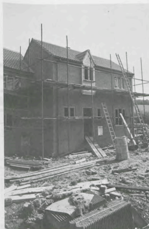
Photo: Northampton Development Corporation
