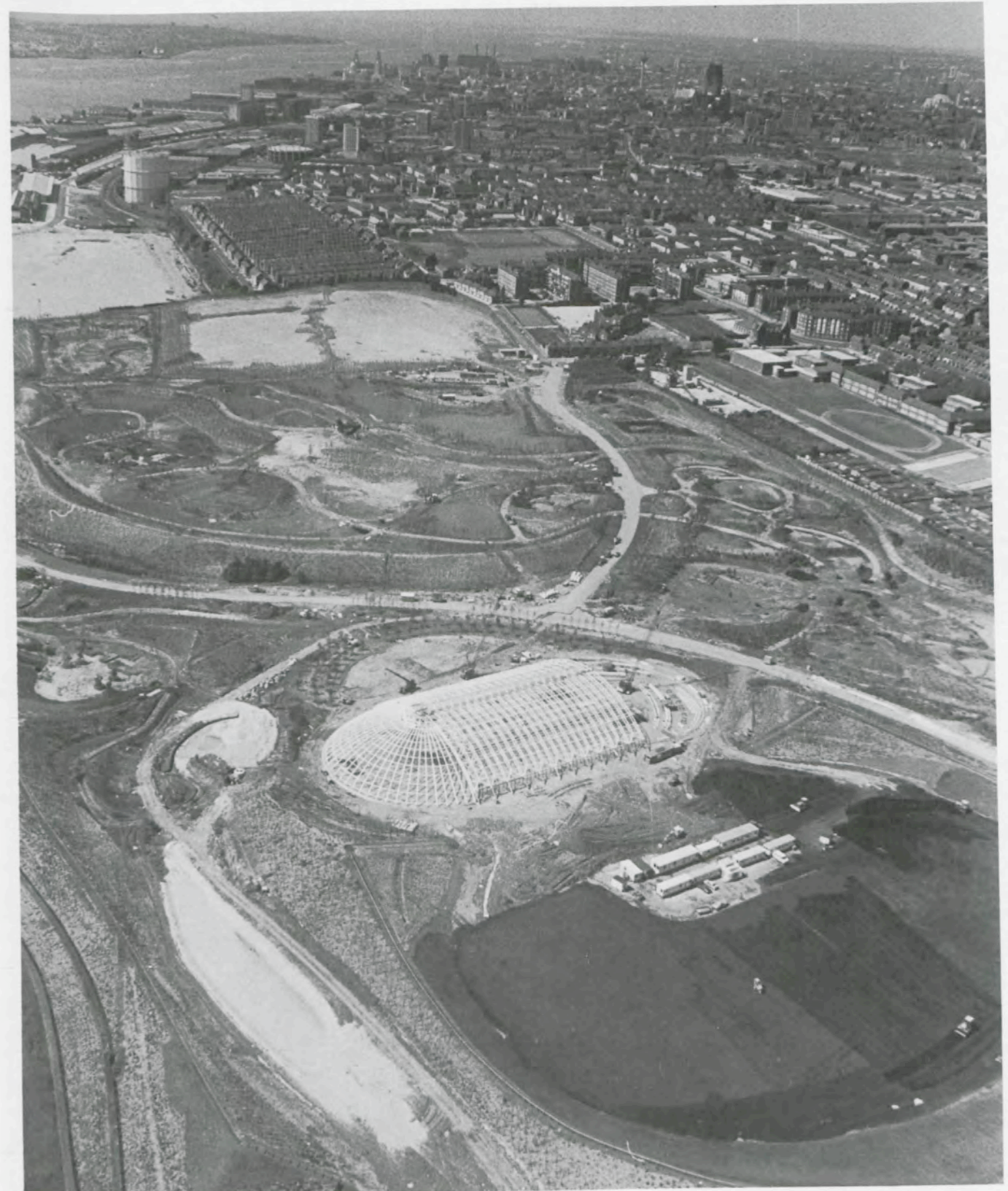
Preparations for Liverpool's 1984 International Garden Festival continued on the site of the former docks. This photograph, taken just after the end of the year, shows the Exhibition Building taking shape.
