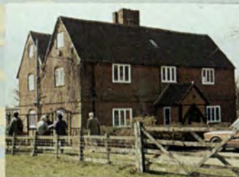
IMAGE HOUSE: AN INTERESTING EXAMPLE OF AN EARLY 18TH CENTURY RED BRICK FARMHOUSE.
