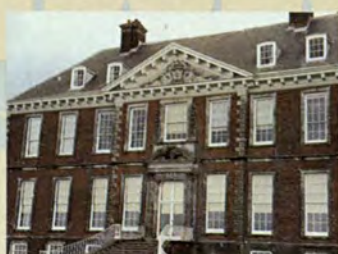
UPPARK: A GRADE I LISTED BUILDING OF EXCEPTIONAL INTEREST ILLUSTRATING THE SURVIVAL OF AN IMPORTANT 17TH CENTURY DESIGN.
