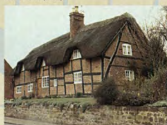
1 BIRMINGHAM ROAD, STONELEIGH, WARWICKS. A TIMBER FRAME AND BRICK COTTAGE RETAINING MEDIAEVAL CRUCK FRAMES AT EACH END.
