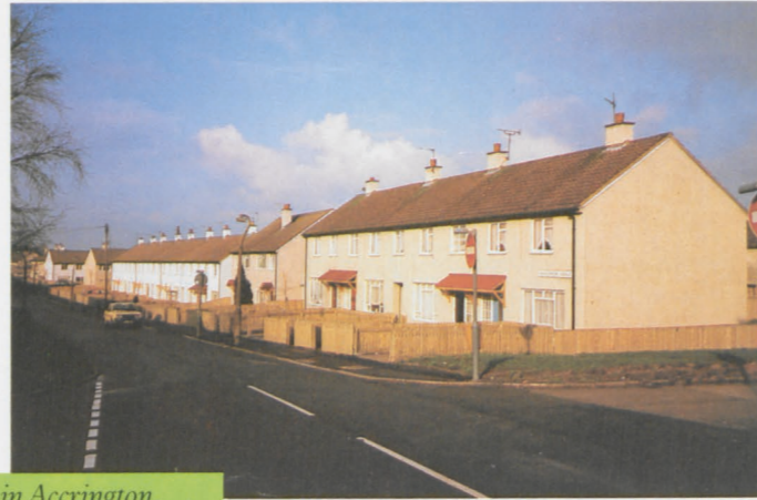
At the Huncoat Estate in Accrington, external cladding to the walls of the houses was provided. This not only makes heating the houses much easier, but also dramatically improves their appearance.
