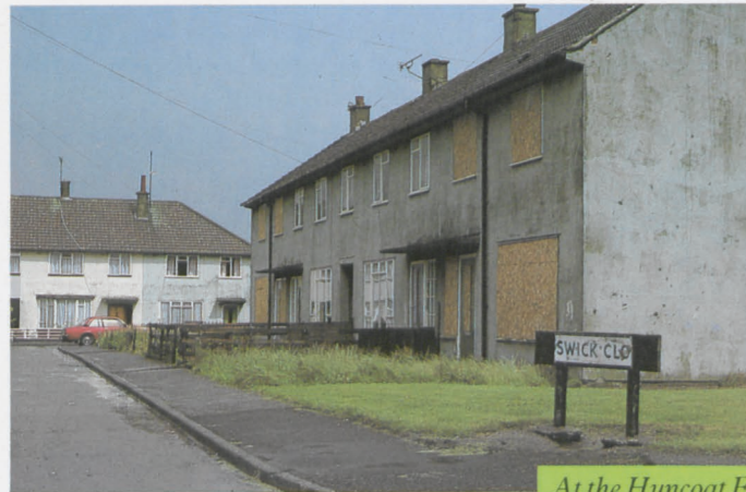
At the Huncoat Estate in Accrington, external cladding to the walls of the houses was provided. This not only makes heating the houses much easier, but also dramatically improves their appearance.
