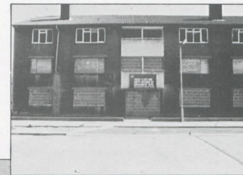
A derelict block at Langridge Crescent prior to improvement.
