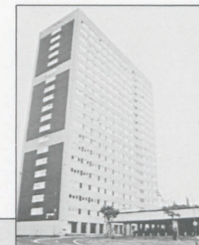
One of the blocks prior to external improvements including demolition of the car park in the foreground.
