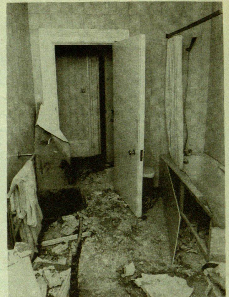
A near thing — the wreckage of Mrs Thatcher's bathroom
