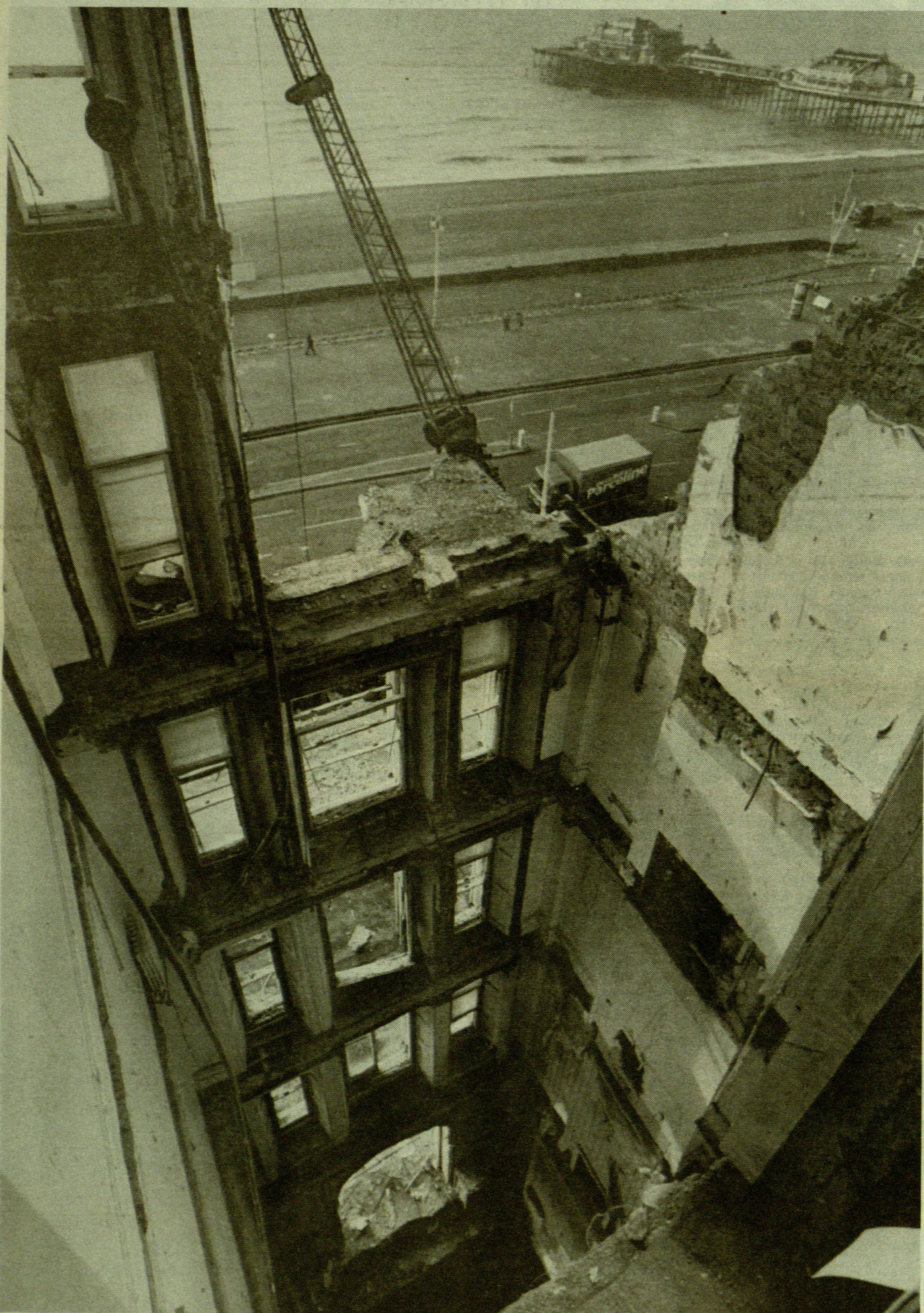
The bombers' legacy — a gaping chasm through the centre of the Grand. It was down this hole that guests on the upper floors hurtled as the chimney collapsed and tilted rooms in a helter-skelter of fear
