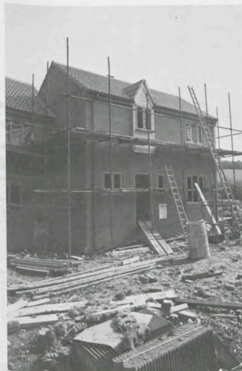
Photo: Northampton Development Corporation
