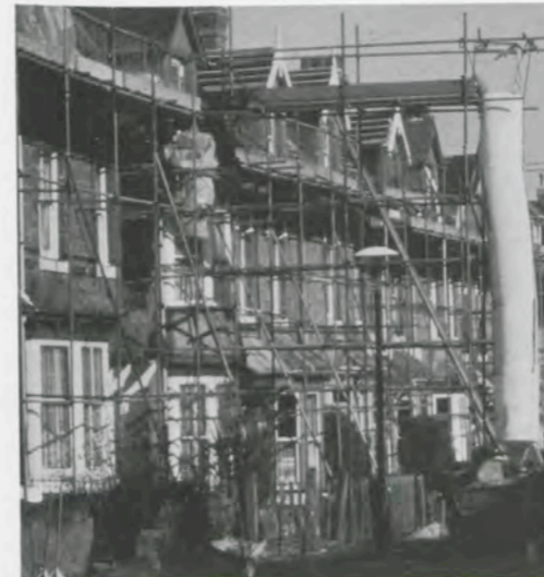
Enveloping, the exterior renovation of whole rows of houses
