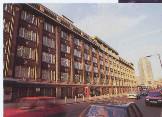
Cornwall House is situated close to the South Bank Arts complex.
