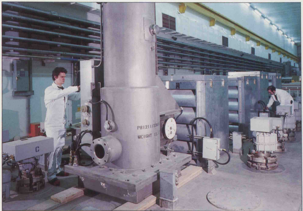
Lower maintenance corridor.
