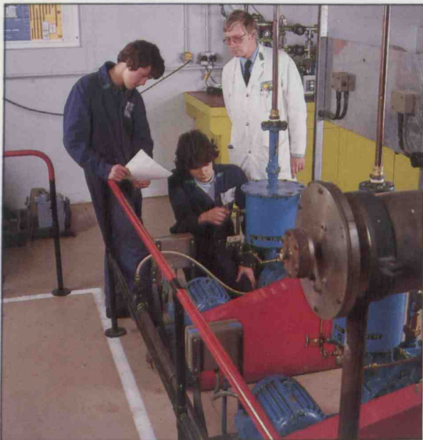
Two fitter apprentices working on a Kinney Pump used in vacuum work.
