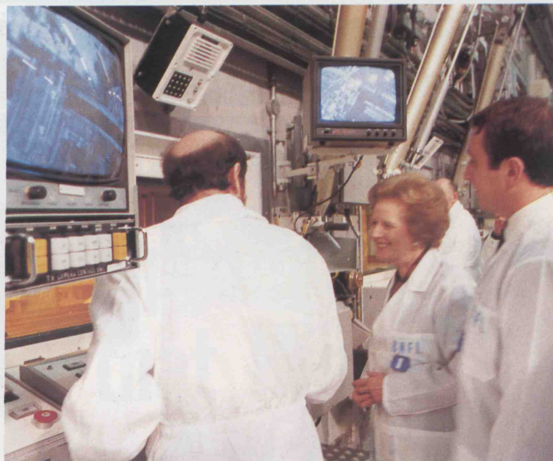
ON THE SCREEN . . . Television cameras give operative Robert Taylor a clearer picture at a decanner control station in the FHP at Sellafield.
